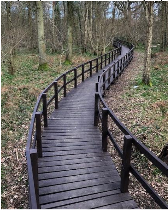
Recycled plastic boardwalk at Wykery Copse, by Creative Timber.
