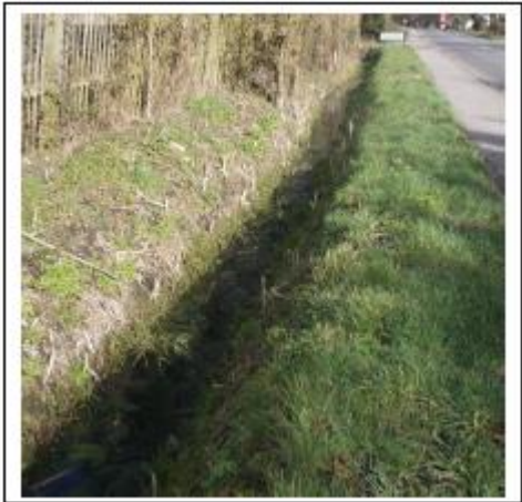
Figure 2: A ditch running alongside the public highway which is the responsibility of the private land owner.
