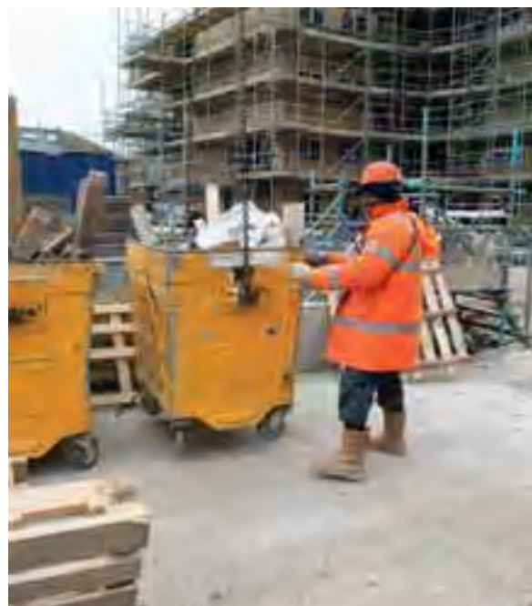
On-site separation of construction waste. Credit: WRAP
